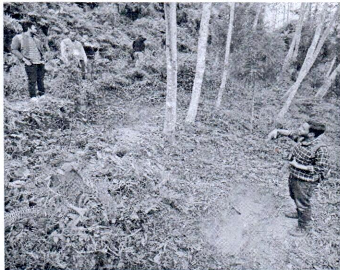
Photo plate 6 Initiative taken (trench excavation for water recharge) under Jharnadhara programme for management of spring water, Sangsey, Kalimpong II block, Kalimpong district
